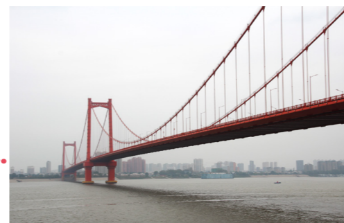
Yingwuzhou Yangtze River Bridge
