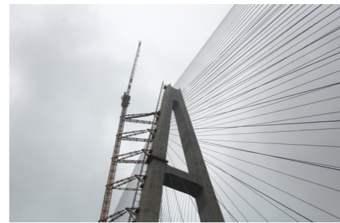
Qingshan Yangtze River Bridge
