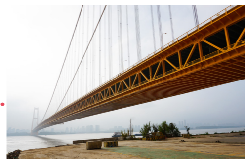
Yangsigang Yangtze River Bridge
