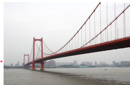
Yingwuzhou Yangtze River Bridge
