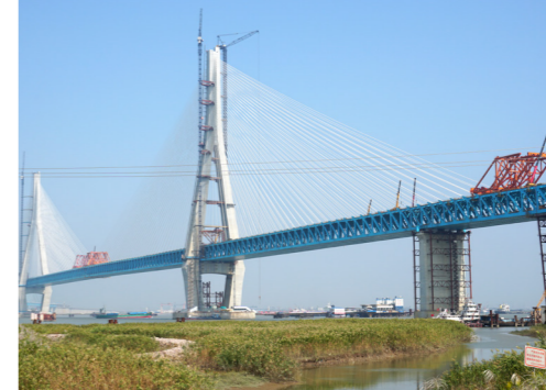
Hutong Yangtze River Bridge Nantong
