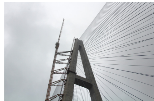
Qingshan Yangtze River Bridge
