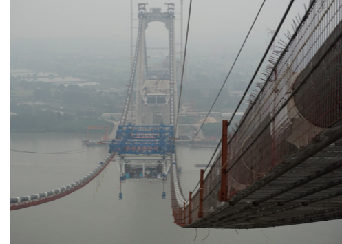
Wufengshan Yangtze River Bridge Zhenjiang
