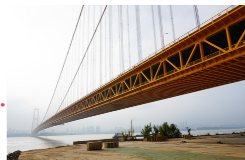
Yangsigang Yangtze River Bridge
