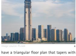
increasing height. This is intended to achieve better stability against seismic interventions and wind events. The triangular shape is based on three large reinforced concrete columns that taper upwards. These columns meet at the top and form a 61 m high crown structure. The dome is made of glass. At some points in the building, slots are built into the building envelope, which should lead to wind load reduction.
